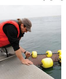
installation of Pickering Nuclear's fish protection net. In its third full year of operation, the Pickering fish net has significantly reduced the volume of fish entering the station's water intake channel.
